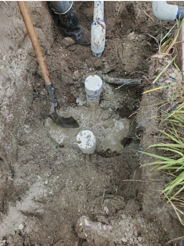
Thrust block installation along north side of Covington Stone.
